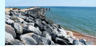
ROCK ARMOUR/RIP RAP
